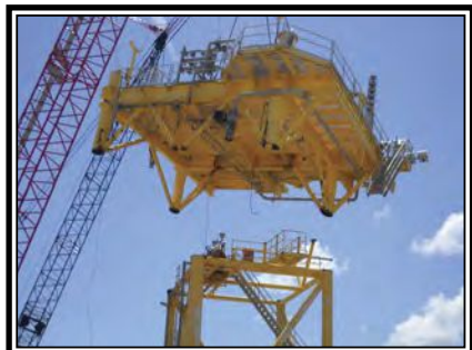
Crane Offloading Structure
